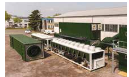
Ventilation and Cooling System for a Shaft Sinking Project, United Kingdom
